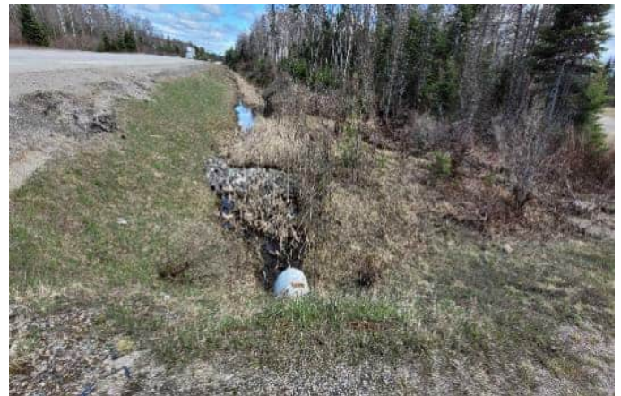
Photograph 48 ↑ Notman –14+926: May 2, 2024. View of upstream ZDA. Facing upstream (southeast) from entrance along ditchline. Perched entrance culvert (Photo 53) and riprap in ditch are both fish passage impediments..
