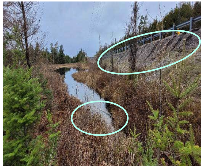
Photograph 26 ↑ Blyth – 15+512: April 30, 2023. View of the downstream ZDA, facing downstream (northwest) along channel to wetland. Embankment erosion is shown, and deposited material was observed in this channel.
