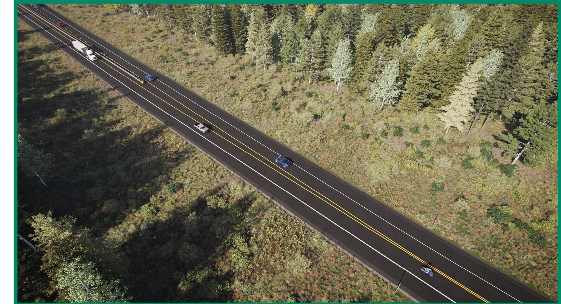
Example of Steel Beam Guide Rail with Start and End Condition Proposed for northern GWP 5033-22-00
